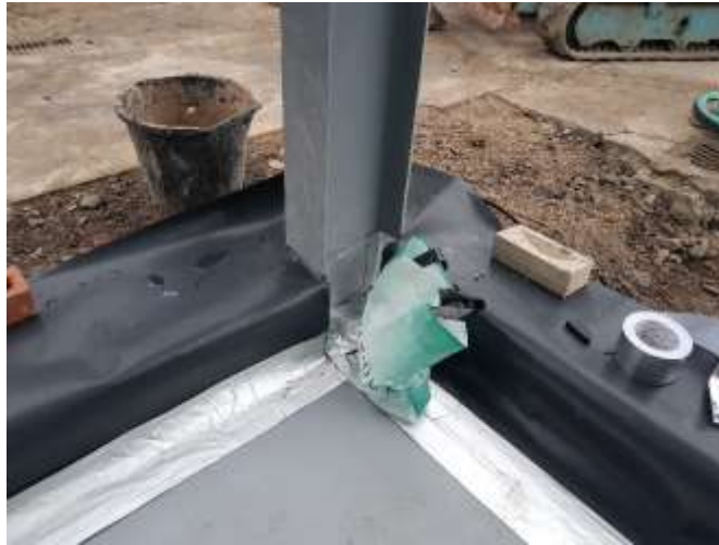
Plate 4: Hydrocarbon Membrane installation around column and up to external wall.
