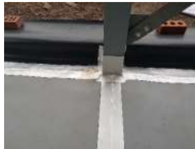
Plate 2: Hydrocarbon Membrane installation around column and up to external wall.
