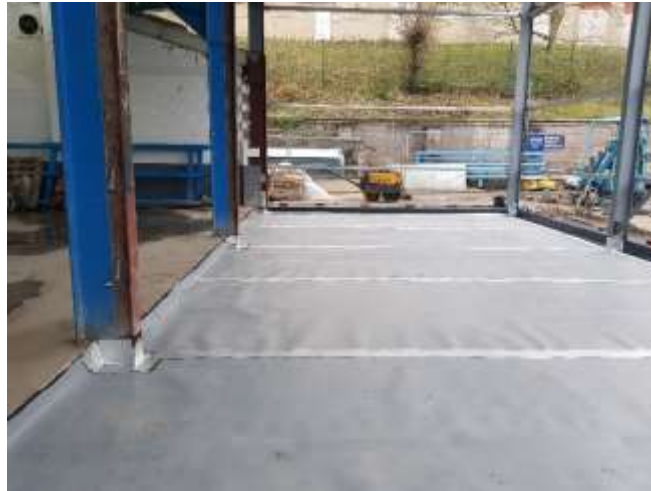
Plate 1: Hydrocarbon Membrane installation across Loading Bay building.
