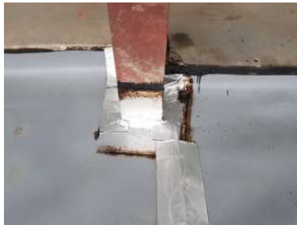
Plate 3: Hydrocarbon Membrane installation around column and up to internal wall.
