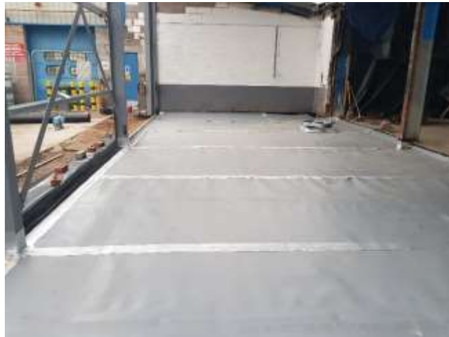
Plate 5: Hydrocarbon Membrane installation.
